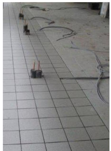
Drainage up stands - must be fully dressed with no exposed screed into which pests can burrow. Where drainage is to a suspended floor, the core-cut hole should be sealed to both sides of the floor to prevent pests accessing any floor cavity that may exist and prevent them moving between floors. Upstands should be fitted with an adapter.
