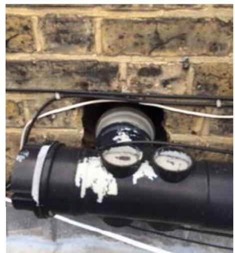
External waste pipe with no seal leaving big entry points.
