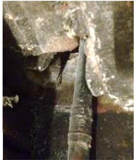
Pipe hole in the brickwork with visible gaps for rodents.
