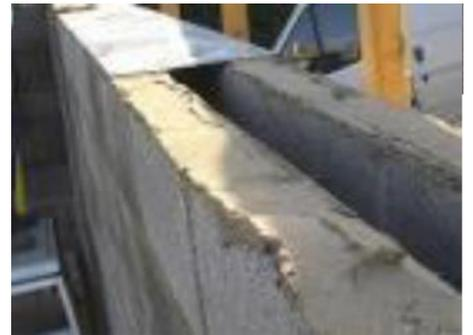
Roller shutters – present a significant risk for mouse ingress. At the closed position there should be no gaps 5mm or greater. Where possible a brush strip should not be used but a combination of rubber boot and proofing blocks.
