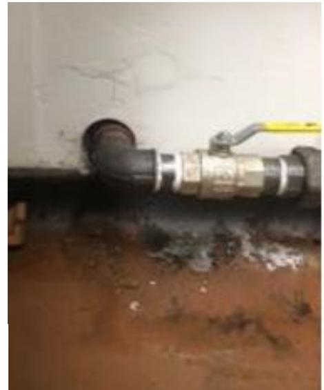
Expanding foam, which has not been used correctly leaving big gaps for rodents to gain entry.
